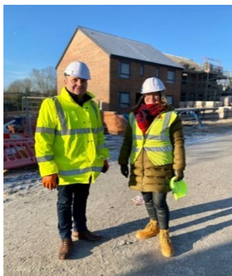
Redditch Council Houses being built in Church Hill
